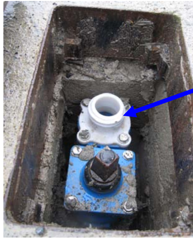
Figure 4.0 – Plastic/nylon outlets on hydrants
